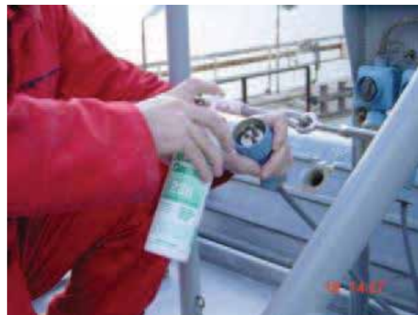
Image 18.b Applying VpCI® 238 for protection of electric contacts
