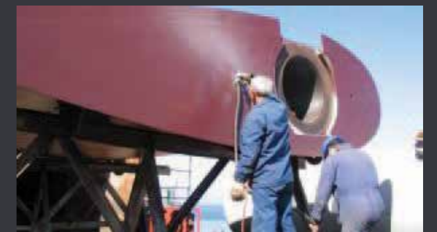
Corrosion inhibitor is blown into the rudder through openings.
