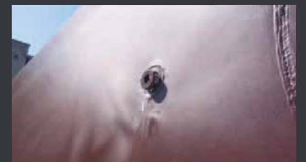
Closing of the opening with the tap. Moving on to the next chamber.
