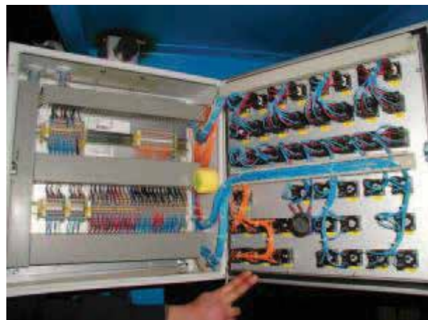
Image 18.a Applying VpCI® Emitter in electric panel
