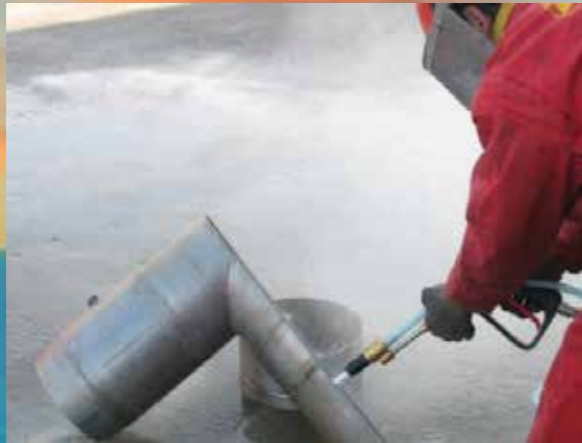
Figure 10. Surface preparation with wet blasting process
